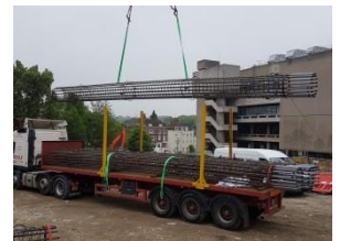
Pile cage delivery
