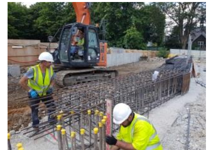
Construction of capping beam
