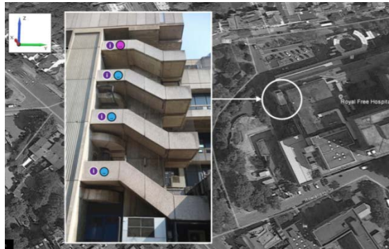
North-West External Concrete Stair
