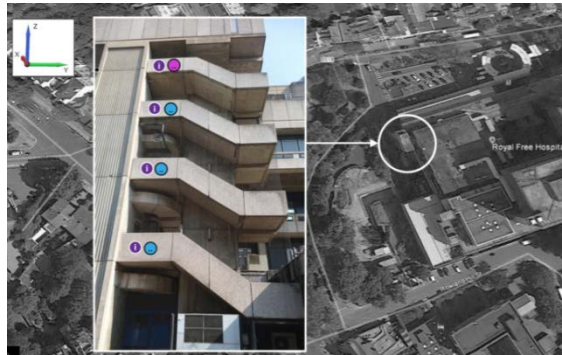
North-West External Concrete Stair
