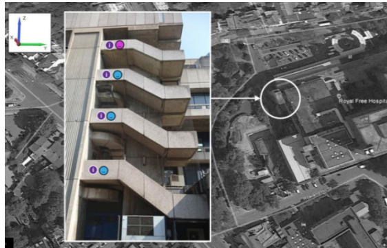
North-West External Concrete Stair
