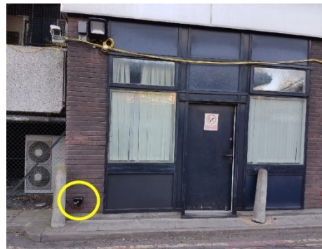
MRI Scanner Room 4
