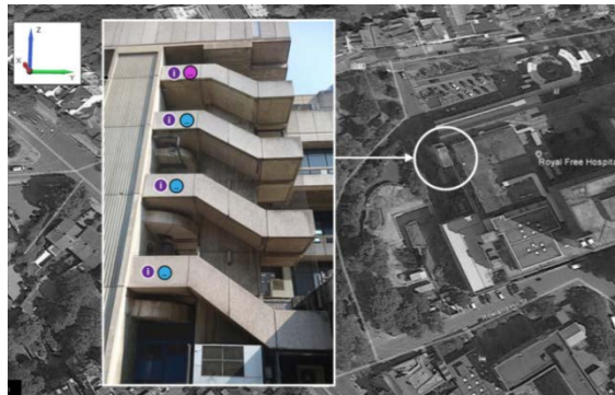
North-West External Concrete Stair
