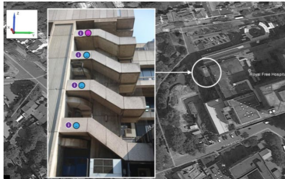
North-West External Concrete Stair
