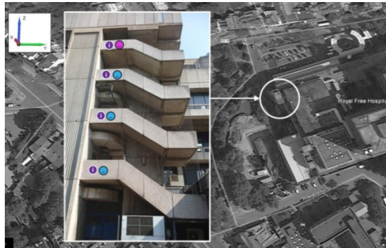
North-West External Concrete Stair
