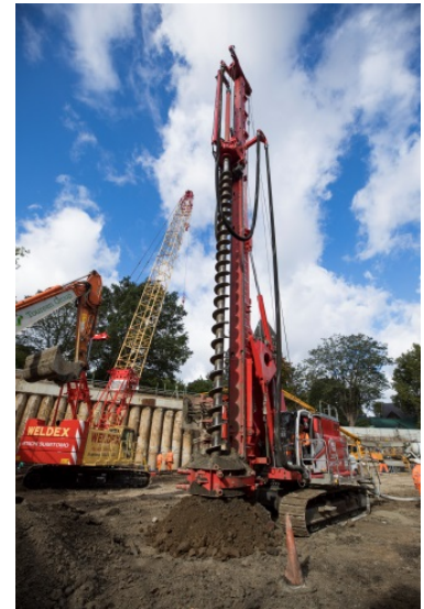
Foundation Piles in progress
