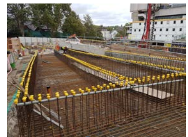
Works to external retaining walls
