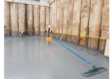
Casting of basement slab
